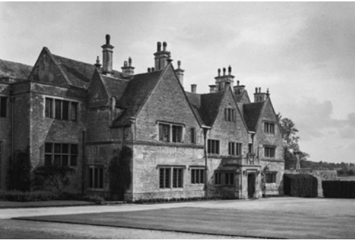
Barnwell Manor, Northamptonshire. © Country Life Picture Library
