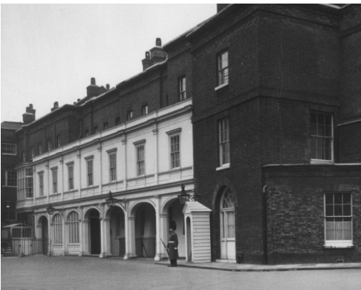
York House, St. James's Palace.
